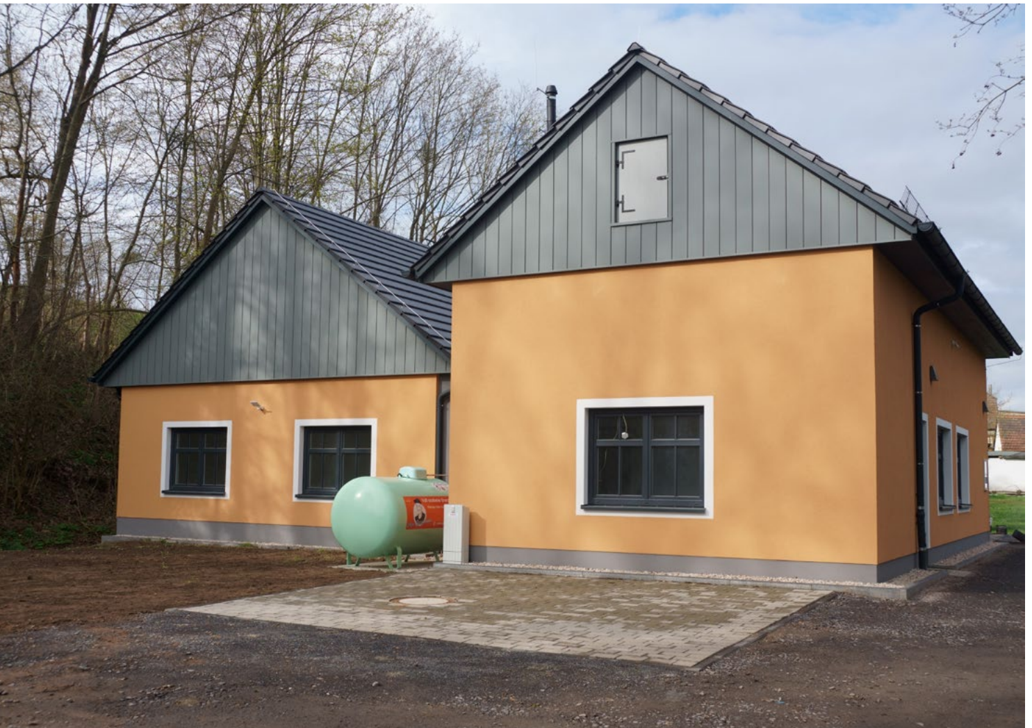
Photo 11: Village community center in the district of Reichardttsdorf with biological sewage treatment plant © Stadt Bad Köstritz
