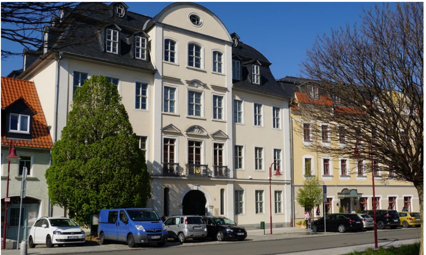
Photo 14: Establishment of a public toilet in the city hall (palace building) © Stadt Bad Köstritz
