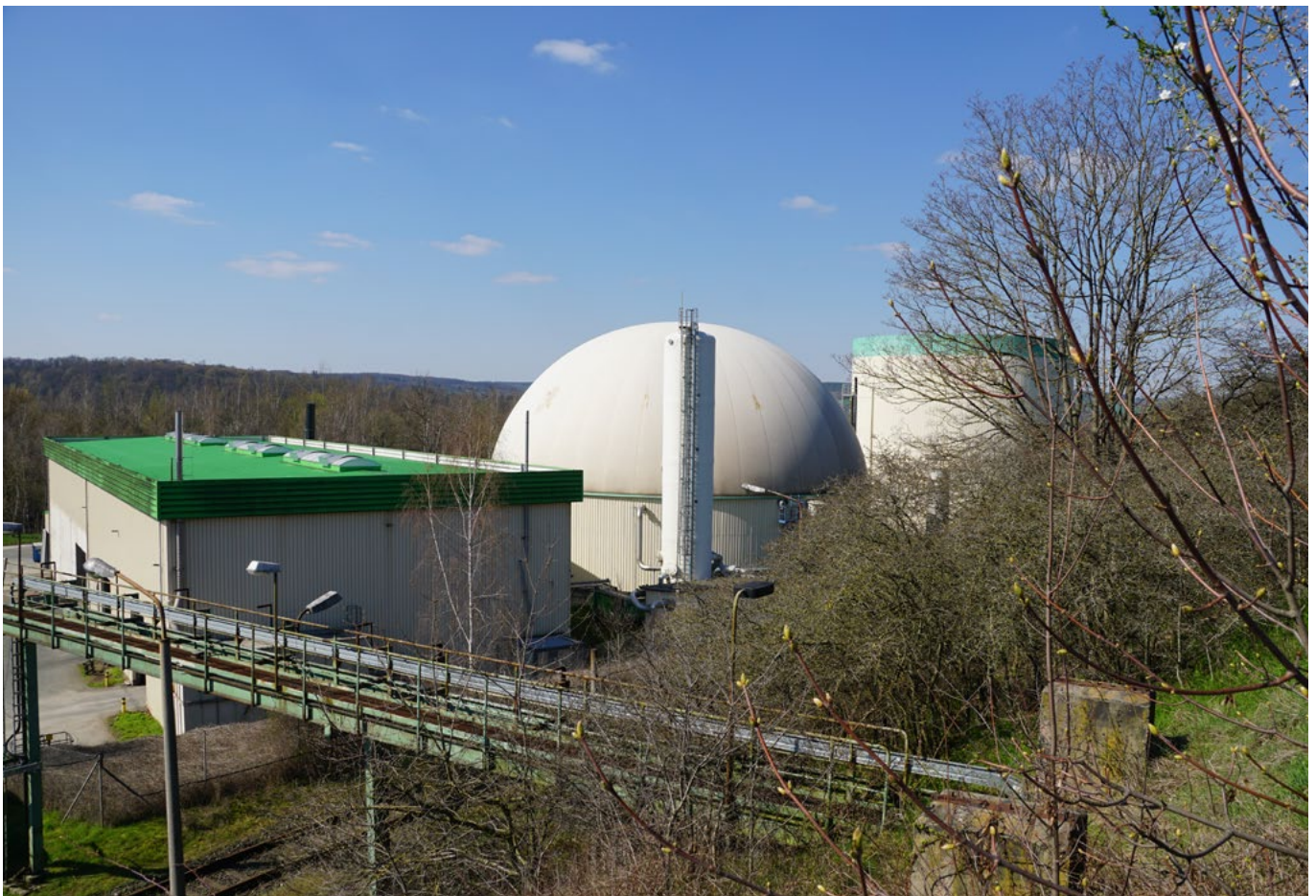
Photo 17: Bioenergy plant © Stadt Bad Köstritz
