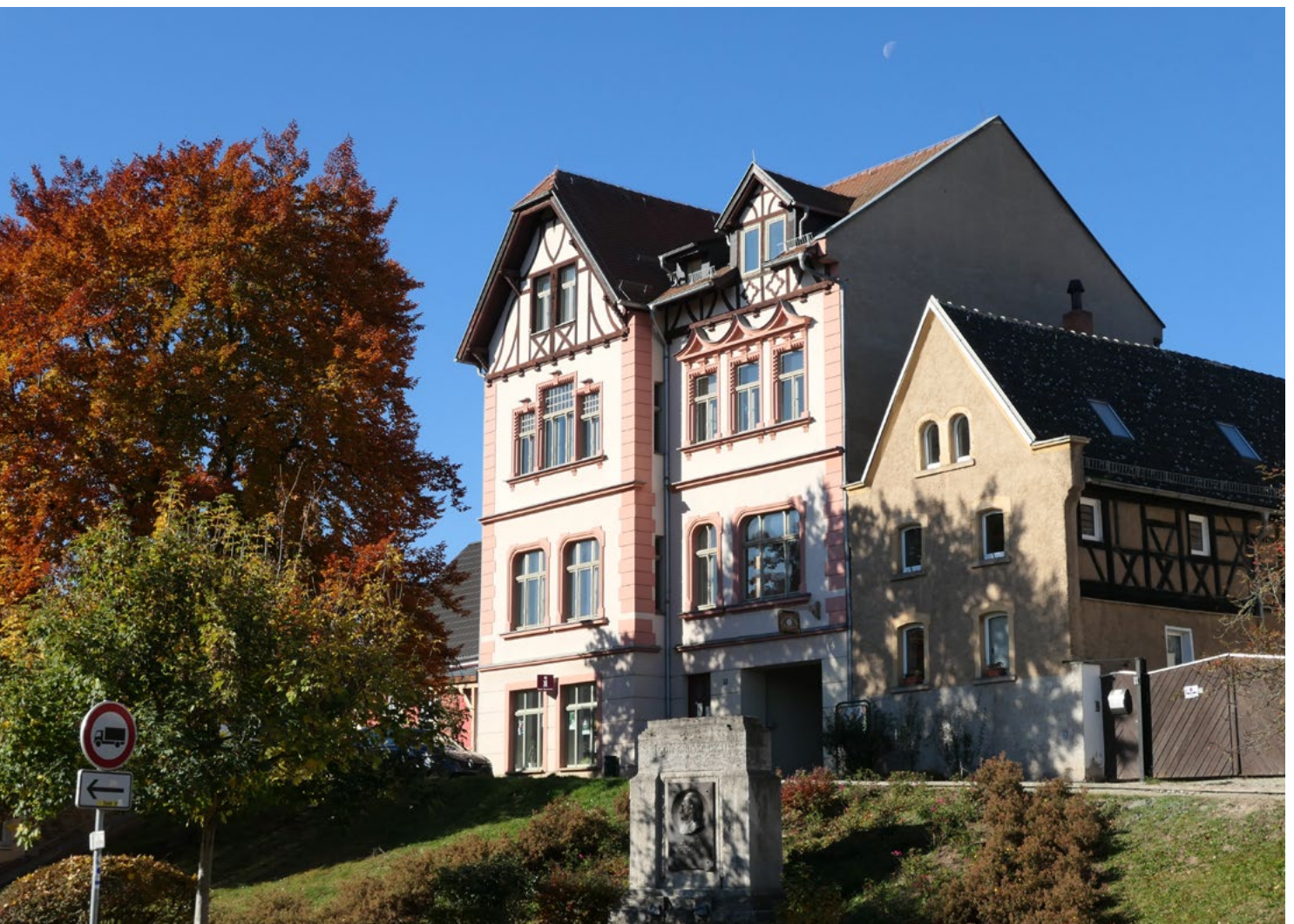
Photo 24: Barrier-free access to the community center "Gucke" in the House of the Guest © Stadt Bad Köstritz
